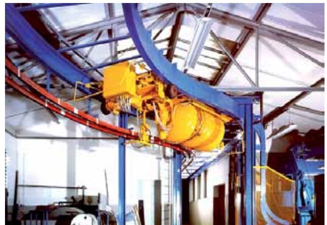
Feed and control of a concrete skipper
