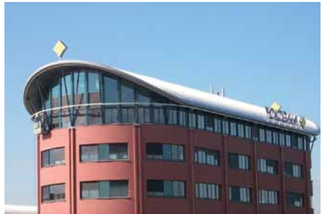
Curved installation for window cleaning equipment
